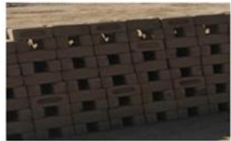
Figure 1.5: Drying of bricks in sunlight.
