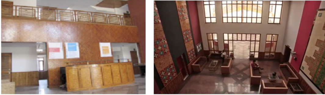
Figure 35: Processed Bamboo board used reception table and wall panelling cladding, staircase and corridor railing Source: Axis Consultants
