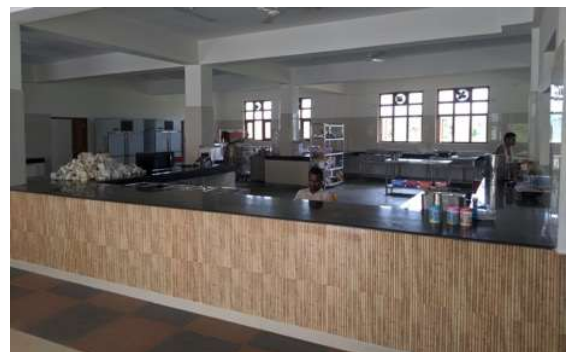
Figure 34: Hollow bamboo used for serving station cladding in the dining hall and for furniture's in the cafeteria .
