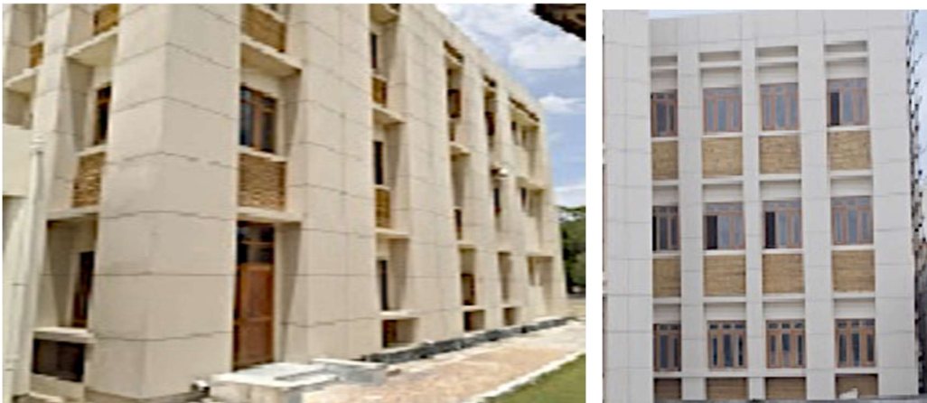
Figure 31: Half-cut hollow bamboo cladding on the external wall Source: Author
