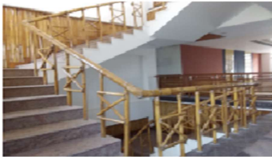
Figure 33: Hollow bamboo used cladding , staircase and corridor railing.
