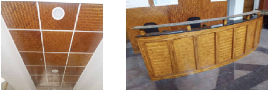
Figure 36: Bamboo mat board for false ceiling and reception table Source: Author
