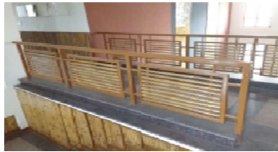
Figure 33: Hollow bamboo used cladding , staircase and corridor railing.
