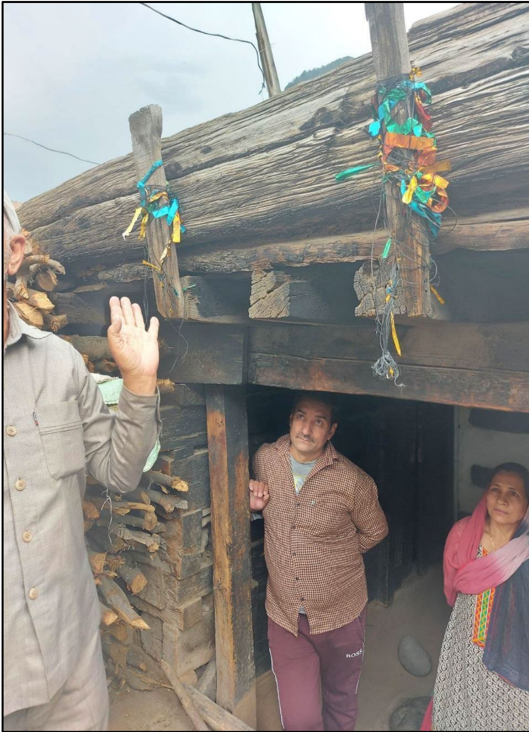
Fig.: 7.34 shows an old traditional house. (source: clicked by scholar)
