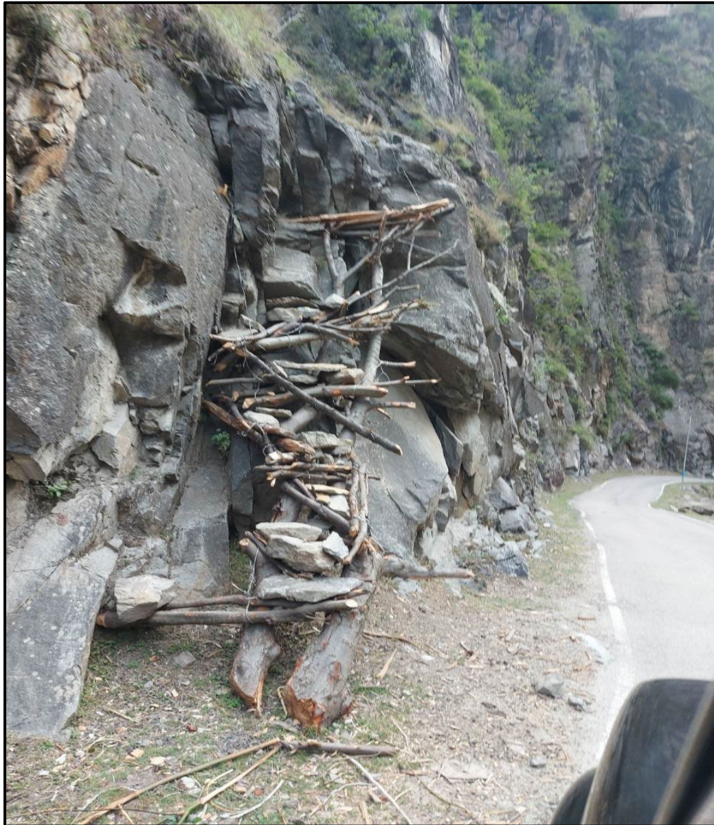
Fig.: 7.35 shows the locally made stair locally known as Taran to collect grass from high reaches. (source: clicked by scholar)
