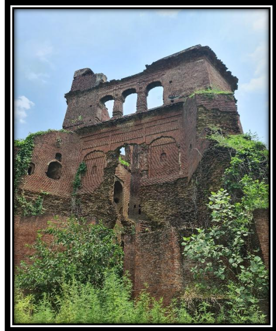
(Plate. 34) East Side Bastion,
