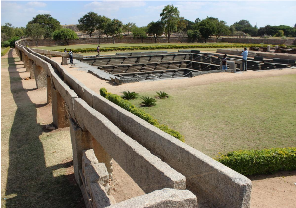
Fig 7: Aqueducts made of stone blocks with slope embankments for water flow (Self Clicked)
